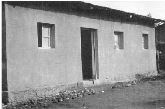
Figure 1: house plastered with lime-pozzolana mix, Rwanda.
