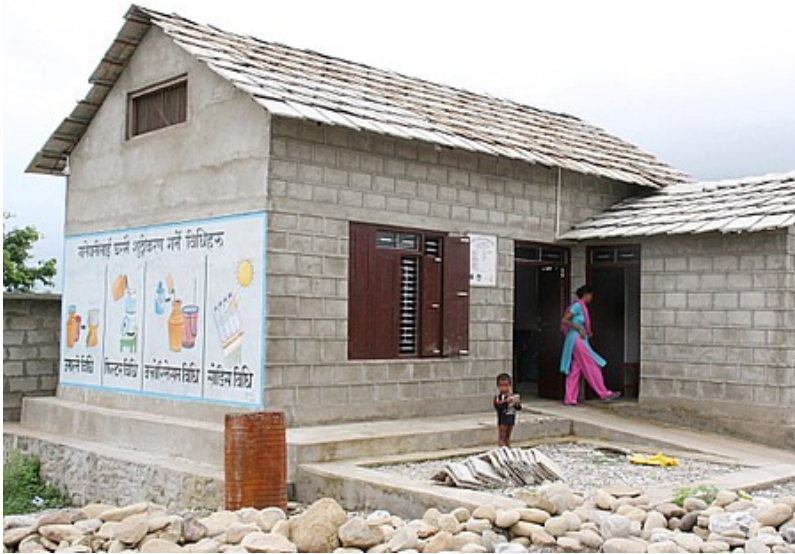
Figure 3: A building of concrete blocks and roof tiles in Nepal. Photo: Practical Action.
