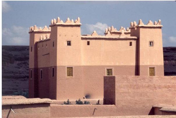
Figure 1: House with stabilised soil render in Atlas Mountains, Morocco. Photo: CRATerre/EAG
