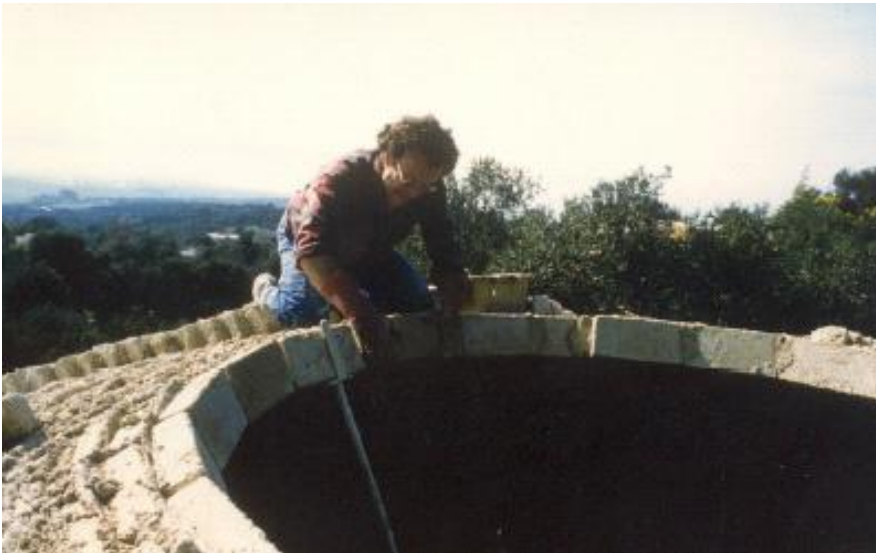
Figure 2: The good cohesion of mud mortar allows construction of vaults and cupolas without shuttering. Photo: CRATerra-EAG.
