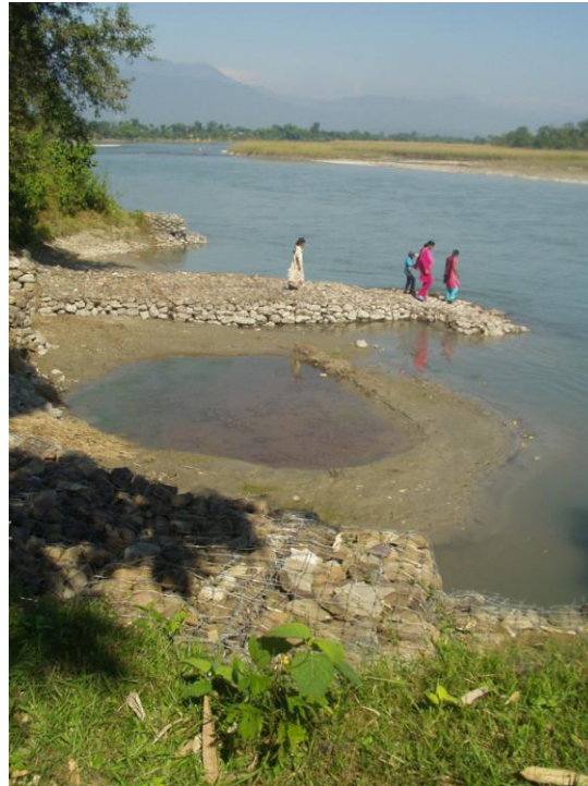
Figure 1: A small spur showing how bank erosion can be reversed by capturing sediment behind the spur. Photo: Practical Action Nepal.
