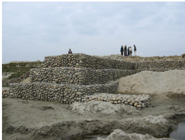
Figure 4: A newly constructed spur shown before the monsoon. The base of the river and the spur apron are clearly visible in the dry season. Photo: Practical Action Nepal.
