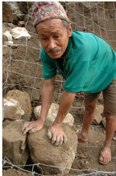
Figure 12: Loading rocks into the gabion cages, a community activity. Photo: Practical Action Nepal.
