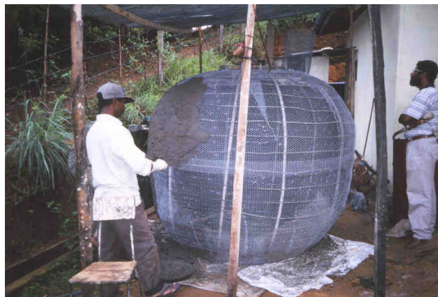
Figure 12: Construction of Pumpkin water tank in Sri Lanka Photo: Practical Action
