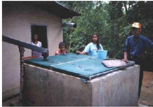
Figure 9: Owner-built RWH storage in post-tsunami Sri Lanka Photo: Practical Action
