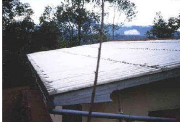
Figure 2: Typical Corrugated Iron Roof, Photo: Practical Action
