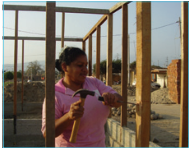
Woman rebuilding a house in Chinchá, Peru, using improved quincha ; this is a relatively simple and familiar technology that self-builders can use with good results
