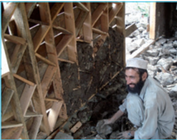
Reconstruction using dhajji dewari , a traditional timber frame wall, filled in with stone and mud, in Kashmir, Pakistan
