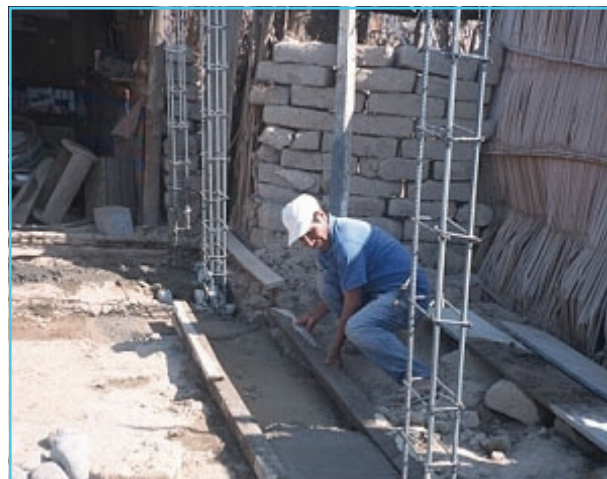
Care needs to be taken to finish the foundations with a perfectly horizontal layer, to provide a good base for the walls
