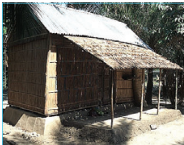
Another rural house in the same country is built on a soil plinth, to lift it above flood waters
