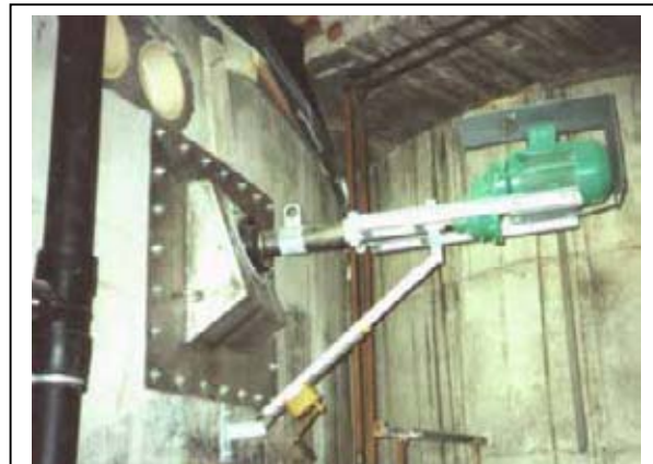
Figure 19: Stirring device for a european biodigester
