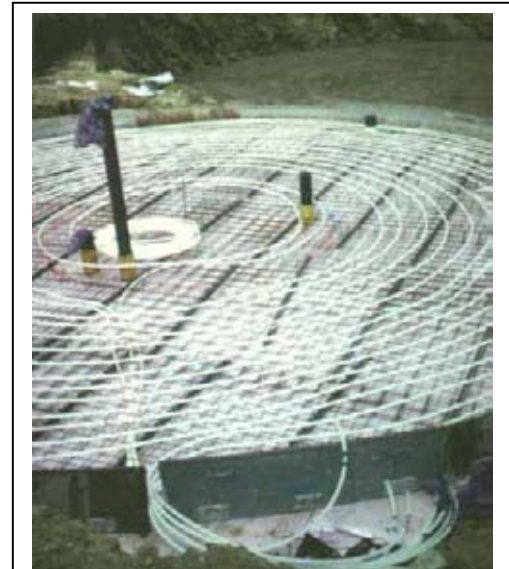
Figure 31: Heating system for a biogas digester under construction (Germany)
