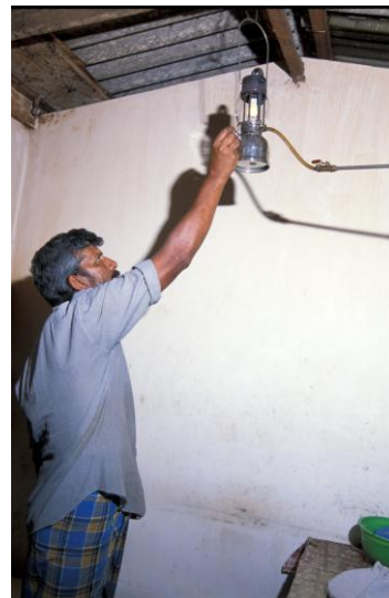
Figure 2: A biogas powered lamp in Bandarawella, Sri Lanka. Biogas is piped directly into the home and used for cooking and lighting. Photo: Practical Action / Zul.
