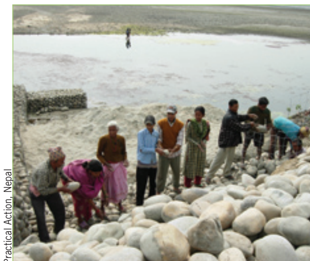
Using gabions to construct dykes for flood protection at Kolhuwa, Nepal
