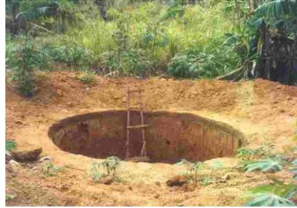
Figure 3: Pit for the tank construction
