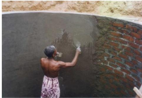
Figure 12: Plastering the tank
